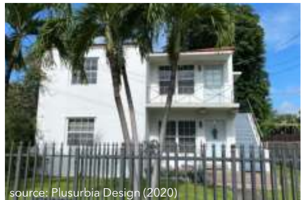
Current photograph of the stacked duplex at 2440-2442 SW 16th Avenue depicted in the diagram above.
