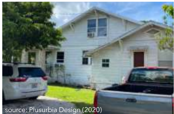
source: Plusurbia Design (2020) Current photograph of the Bungalow at 1710 SW 24th Street, featuring front-facing nested gables with original cedar shingles, wide overhangs, wood siding, and oolitic limestone columns.
