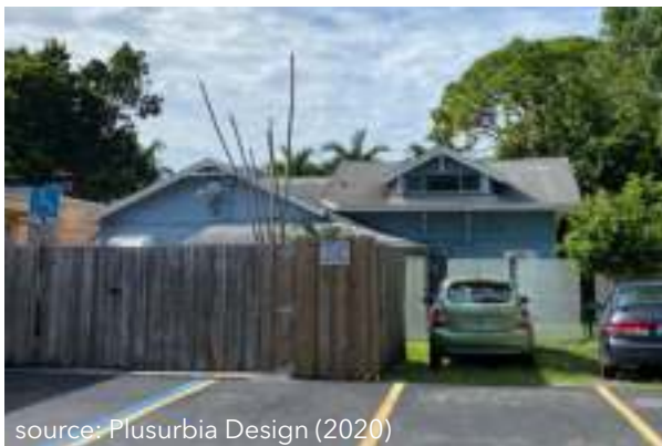
source: Plusurbia Design (2020) Current photograph of the Bungalow at 2287 SW 17th Avenue, featuring a gable roof with overhanging eaves and brackets, a gable dormer, and simple, wood frame construction.
