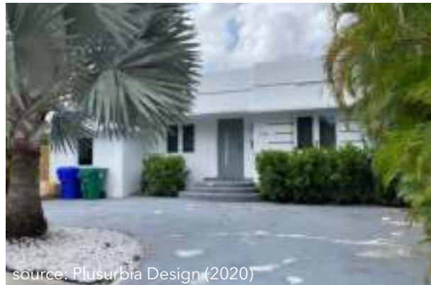
Current photograph of the Moderne-style residence at 2451 SW 23rd Terrace in Silver Bluff, featuring strong horizontal lines, a continuous eyebrow overhang, scored stucco, linear grouped scuppers, and vertical fluting around the front door.
