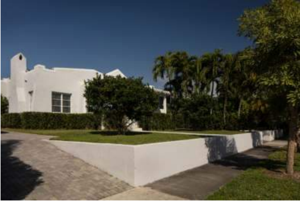
Figure: Elevated properties in Silver Bluff on SW 23rd Terrace, at around SW 23rd Avenue. Source: ©Steven Brooke Studios, Inc.
