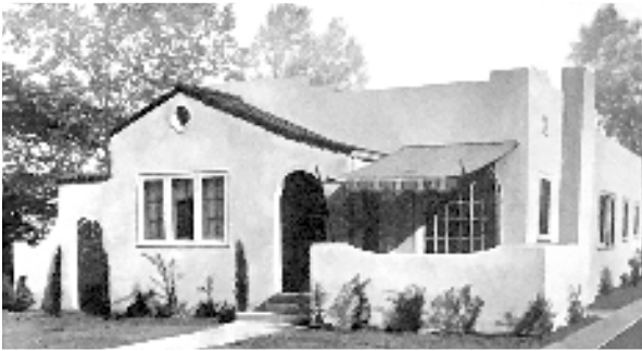
1925 Spanish Cottage. Plan No. 861, Spanish Bungalows , The Bungalowcraft Co., Copyright Rex D. Weston.
