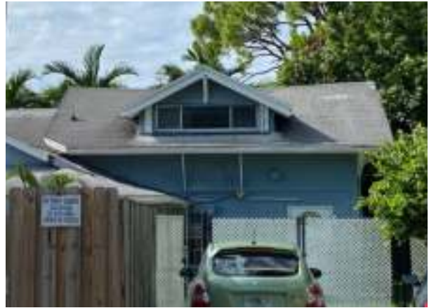
Figure: 2020 photograph of bungalow at 2287 SW 17th Avenue, located behind a restaurant. Source: PlusUrbia Design.
