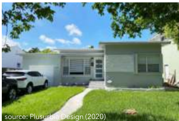
Current photograph of the Mid-Century Modern-style residence at 2387 SW 23rd Street in Silver Bluff, depicted in the diagram above.
