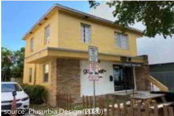
Current photograph of the stacked duplex in the Mid-Century Modern style at 1312 SW 22nd in Silver Bluff featuring a rectangular form, wide roof overhangs, cladstone cladding, and an exterior stairway.
