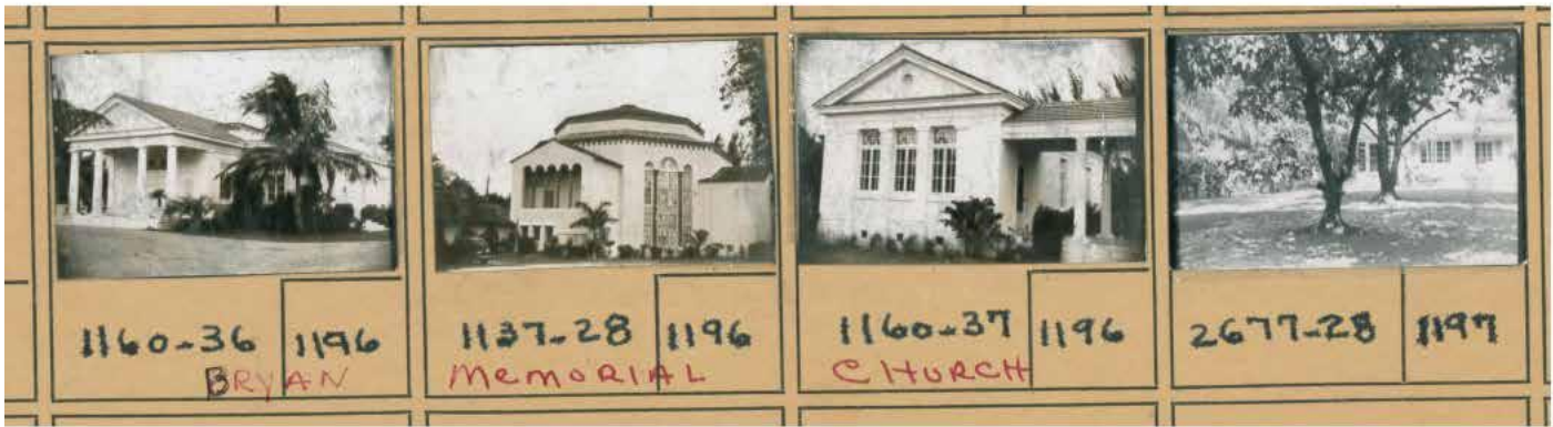
City of Miami, Florida Historic Preservation Office Tax Card
