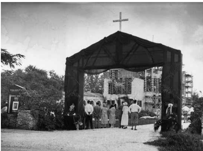
ABOVE: Church under construction ( Miami Daily Metropolis , August 29, 1935)
