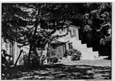
RESTORE OR RAZE? A proposal earlier this year had the 1920s-era house being razed to make way for new homes. A new, but still tentative, plan would have it restored and occupied.
