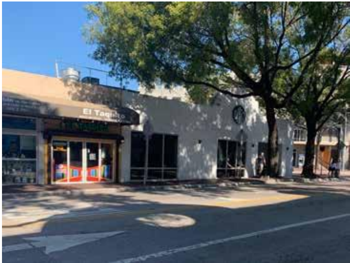
View of Sunshine Building from Main Highway, July 2020. (Kolaya)
