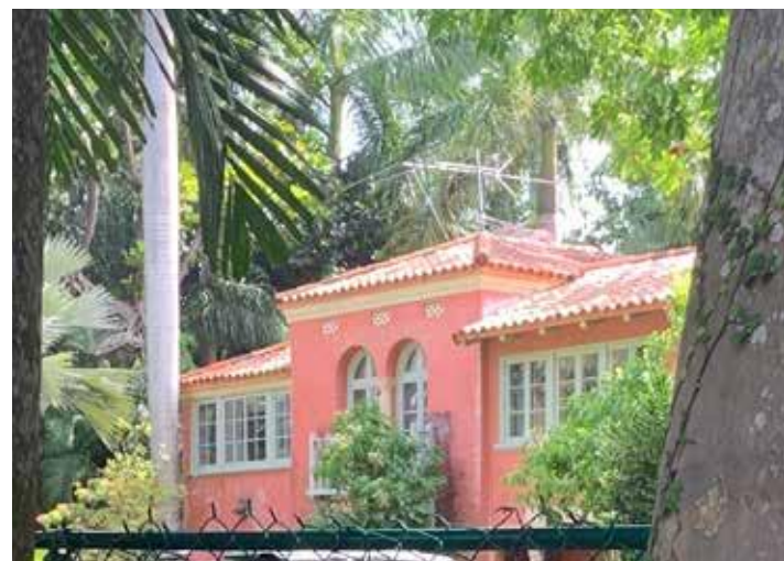
Front façade visible from Hibiscus Street. (Kolaya)
