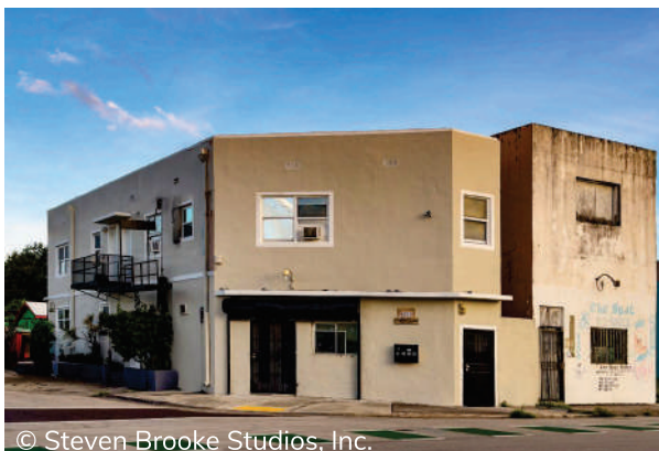
This commercial structure at 6300 NW 15th Avenue was built in 1948 by Hider R. Davie, a wealthy Black businessman who lived at 6595 NW 17th Ave. It is a small commercial block typical of 15th Ave. in Liberty City.
