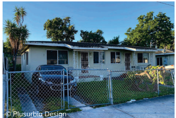
© Plusurbia Design This one-story Ranch-style duplex at 1536 NW 71st Street was built c.1958 and features a broad form with a symmetrical façade with projecting front porches under main roof shed extensions.
