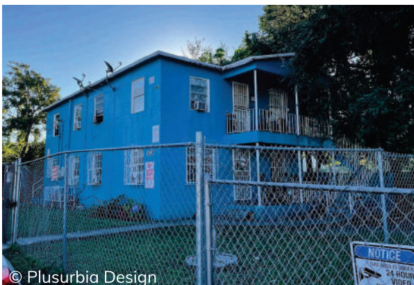
This Masonry Vernacular duplex at 1439 NW 68th Street was built in 1948 by S.C. Chandler. The building features a pedimented two tier porch and horizontal scored stucco lines.
