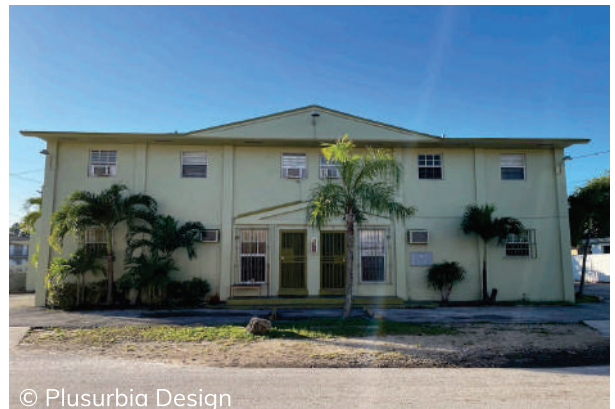
© Plusurbia Design This two-story Neo-classical Revival apartment building at 1500 NW 69th Terrace was built c.1962. The symmetrical building features a side gabled roof, a centered entrance with a pediment and pilasters, and a rear exterior staircases.
