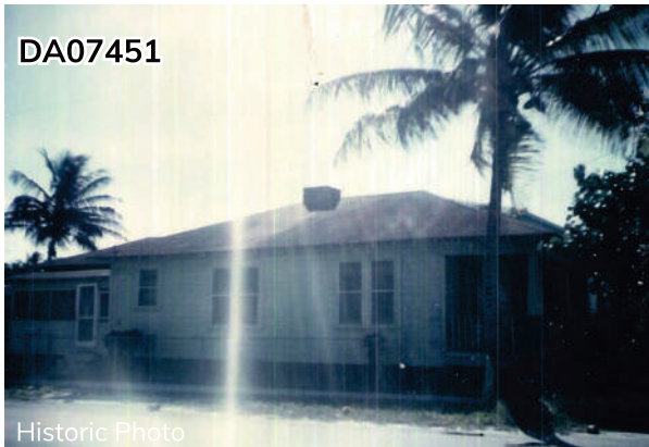
HIDER DAVIE'S RESIDENCE ADDRESS: 6595 NW 17 AVE YEAR BUILT: C.1939 STYLE: CRAFTSMAN ELIGIBLE FOR NRHP DISTRICT
