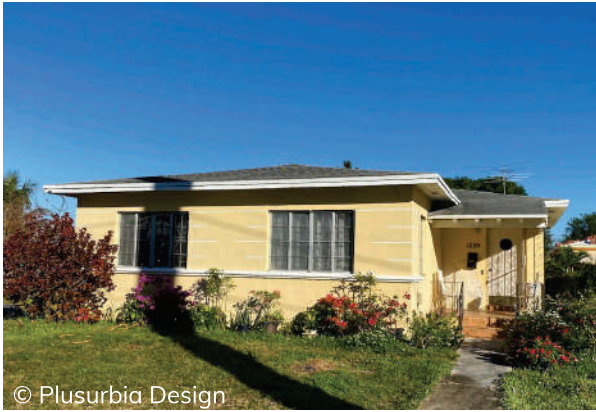
This Ranch-style house was built in 1949 at 1235 NW 67th Street by Miriam Stirrup and William Stirrup, a mail handler at the post office. The house features a recessed attached garage and a recessed open corner entry porch with a shed roof and exposed roof rafter tails.
