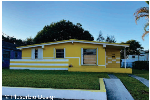
This one-story Mid-Century Modern house was built c.1959 at 1386 NW 71st Street and is notable for its low-pitched gable roof with wide overhangs, exposed roof beams, and the corner front porch with an obscured entrance.
