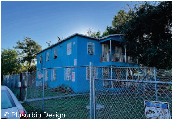
© Plusurbia Design This Masonry Vernacular duplex at 1430 NW 68th Street was built in 1948 by S.C. Chandler. The building features a pedimented two tier porch and horizontal scored stucco lines.
