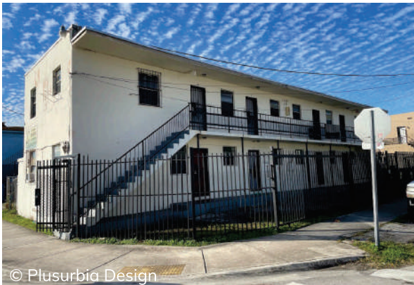
© Plusurbia Design This two-story, eight-unit, Mid-Century Modern apartment building at 1500 NW 65th Street was built c.1953 and features a flat cantilever roof above the entrances, an exterior staircase on either side of the façade, and a second-story balcony.
