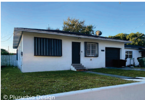
This Ranch-style house was built in 1949 at 1358 NW 71st Street. The house features an attached garage, picture window, and a concrete stoop.
