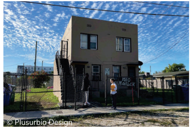
© Plusurbia Design This Moderne triplex was built at 1510 NW 65th Street in 1948 by Willie Mae and Isaiah Williams, who lived there until the 1970s. The building features a flat roof and flat cantilever canopies above the entrances.
