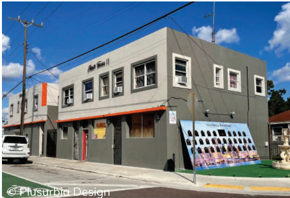
This c.1950 mixed use building at 6829 NW 15th Avenue contained the Jack Thomas Fish and Poultry Market. The building features two stories with a flat roof and concrete eyebrows.
