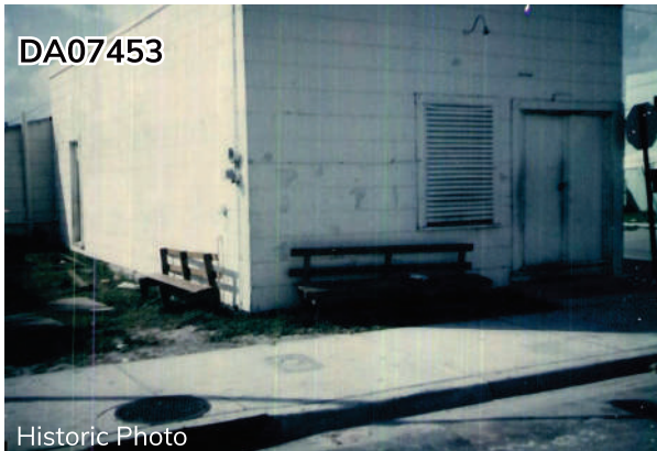
JAMES E. SCOTT COMMUNITY ASSOCIATION ADDRESS: 6248 NW 15 AVE YEAR BUILT: C.1945 STYLE: MASONRY VERNACULAR ELIGIBLE FOR NRHP DISTRICT
