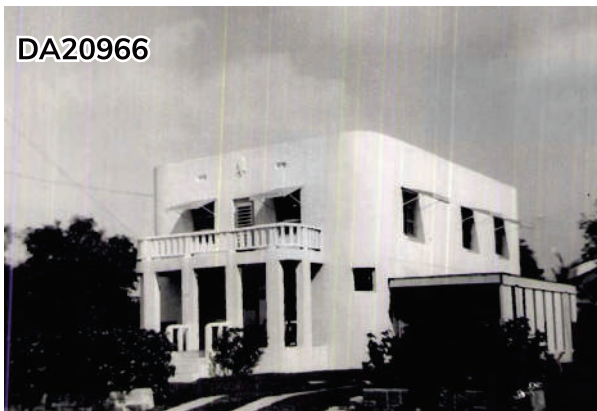
ELDER THOMAS J. RICHARDSON BUILDING ADDRESS: 1353 NW 67 ST YEAR BUILT: C.1947 STYLE: MODERNE ELI
