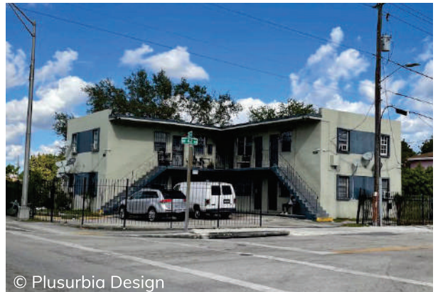
© Plusurbia Design This two-story apartment building at 6251 NW 17th Avenue was constructed in 1956 and consists of ten apartment units. The building features flat concrete overhangs, exterior stairways with decorative railings.
