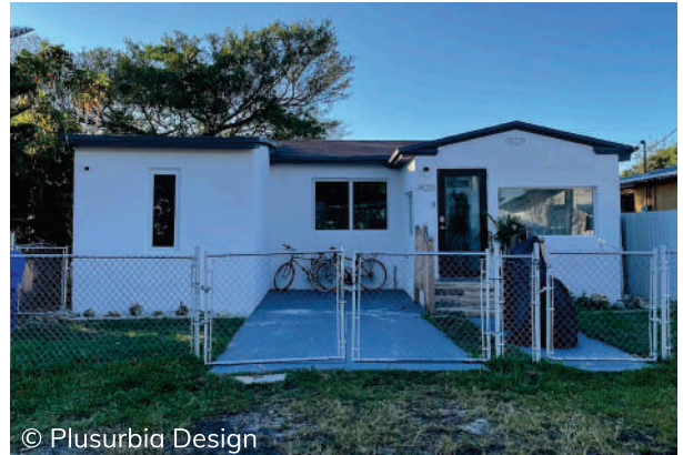
This one-story Minimal Traditional house was built in 1947 at 1420 NW 68th Terrace and features an attached garage and open front entry porch that have since been enclosed. The porch intersecting the gable roof contains a decorative vent motif.
