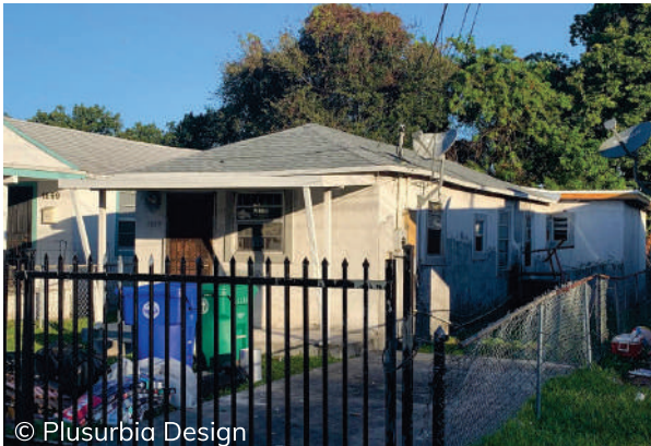
This one-story Frame Vernacular house at 1559 NW 70th Street was built c.1926 and was likely moved to Liberty City in the late 1940s. The original wood siding was replaced with stucco.
