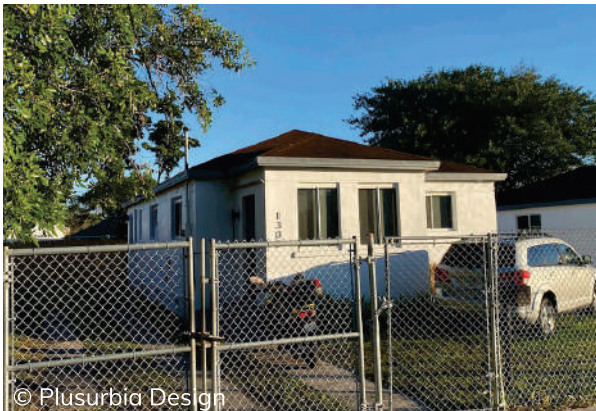
This Minimal Traditional house was built c.1947 at 1305 NW 70th Street and was the residence of Carl Prince. The house features simple and compact massing, a closed projecting front porch with a hip roof, and horizontal stucco scoring aligned with windows.
