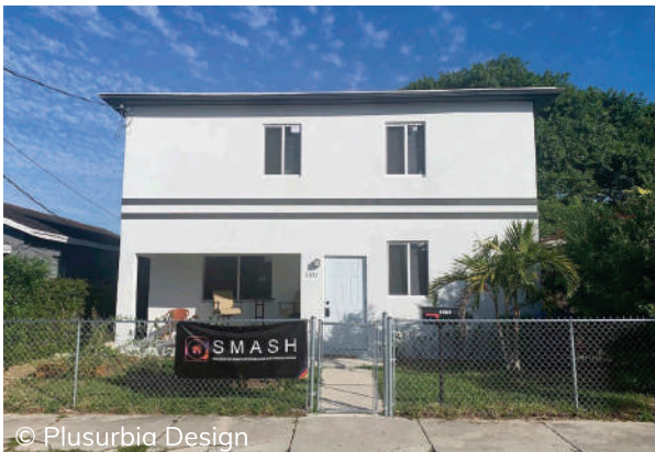
© Plusurbia Design This two-story Streamline Moderne-style duplex was built at 1611 NW 65th Street in 1951 and was the residence of Roxie W. Ward. It features a low-pitch hip roof, wide overhangs, an open incised corner terrace, and a stucco stringcourse.
