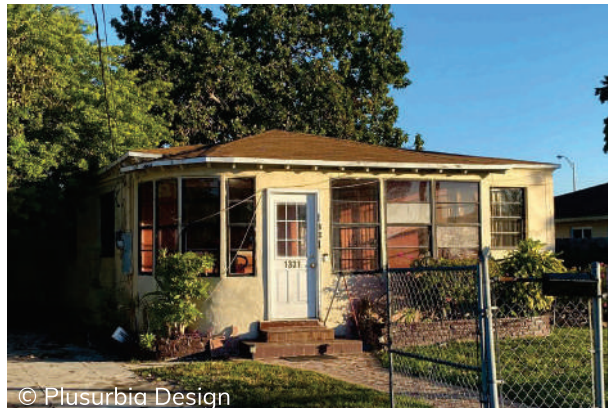
© Plusurbia Design This Minimal Traditional house was built c.1946 and was the home of Mrs. Evelyn and Mr. Clarence Boggs. The house features an enclosed front porch with hip roof and exposed rafter tails and a curved wall. The roof clay tiles were replaced with asphalt shingles.
