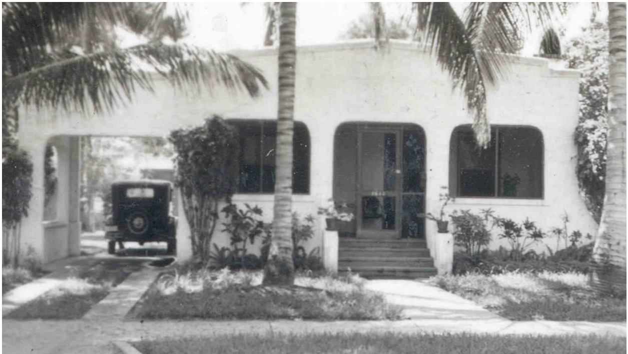
Figure 2.105: Historic photograph of a Spanish-style Bungalow at 1612 SW 11th Street built in 1922 (source: City of Miami, Florida Historic Preservation Office Tax Card Photographs).
