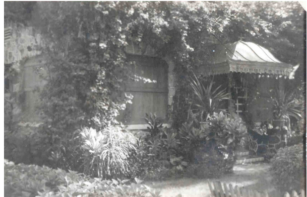
Figure 2.18: Historic 1930s tax card photograph of 1625 SW 12th Street, the original pump house at Shenandoah (source: City of Miami, Florida Historic Preservation Office Tax Card Photographs).
