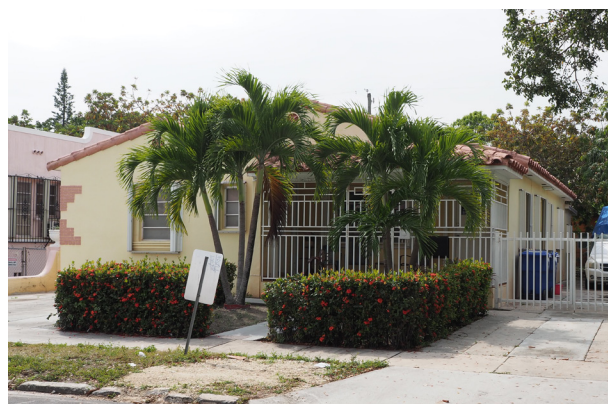
Figure 2.60: Current photograph (2019) of a home in the Minimal Traditional style at 1844 SW 10th Street (source: Plusurbia Design).
