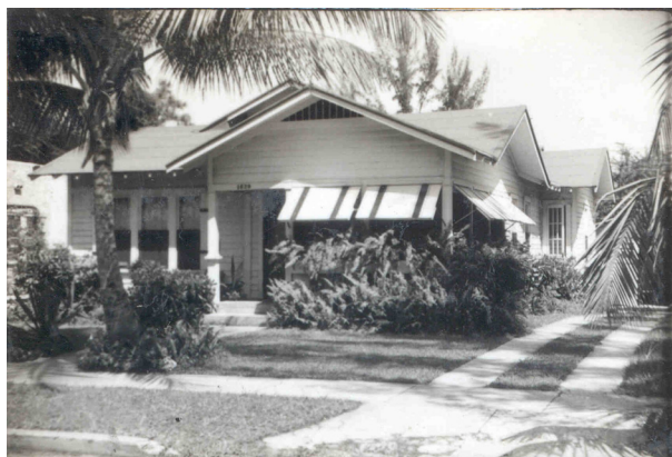
Figure 2.98: Historic photograph of a Bungalow with a porch that has since been enclosed at 1629 SW 11th Terrace (source: City of Miami, Florida Historic Preservation Office Tax Card Photographs).
