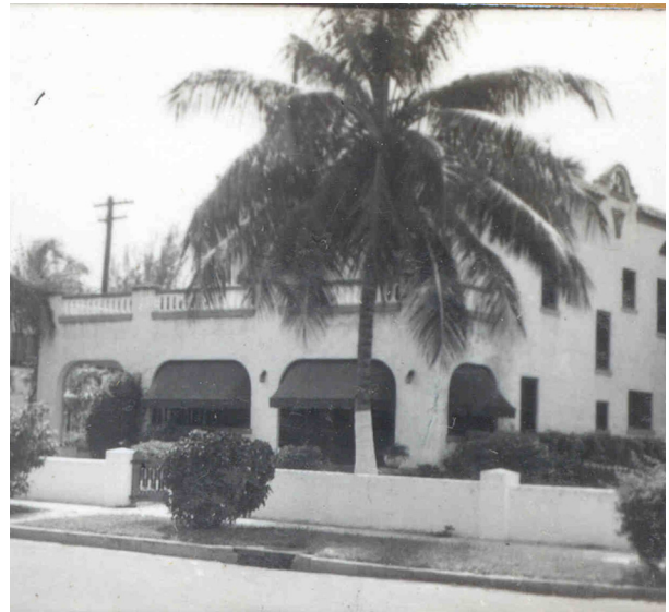
Figure 2.128: A photograph of the residence at 1004 SW 16th Avenue (source: City of Miami, Florida Historic Preservation Office Tax Card Photographs), an example of a Mission-style Kit home.
