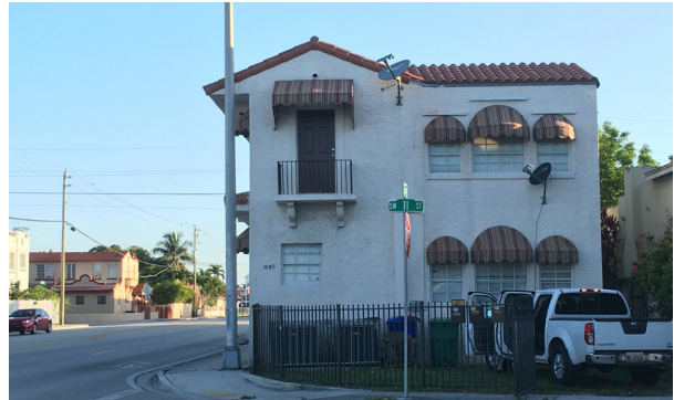
Figure 3.74: Current photograph (2019) of the building at 1695 SW 11th Street. After road widening on SW 17th Avenue, the swale, side yard, and landscaping was eliminated and the residence partially demolished (source: Plusurbia Design).
