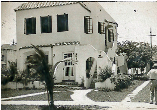
Figure 2.135: Above, a historic photograph of 1872 SW 9th Street residence, one of the 1937 Mediterranean Revival stacked duplexes (source: City of Miami, Florida Historic Preservation Office Tax Card Photographs).
