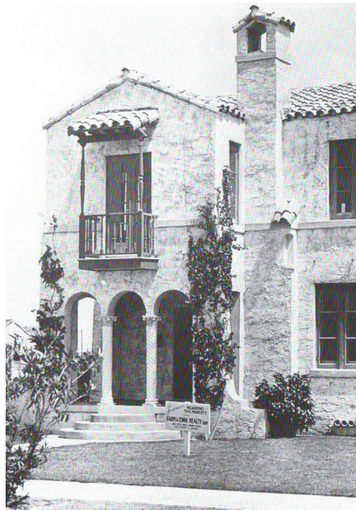
Figure 2.149: Historic photograph of Quinn House, a home in Miami Shores designed by Marion Manley with similar features as 1621 SW 11th Street in Shenandoah (source: Lynn, Catherine and Carie Penabad. Marion Manley: Miami's First Woman Architect . Athens, University of Georgia Press, 2010).
