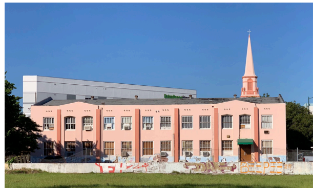
Figure 2.56: Photograph of the building adjacent to Shenandoah Presbyterian Church (source: Flickr user Philip Pessar).
