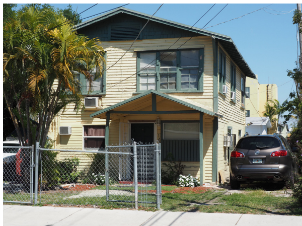
Figure 2.85: Current photograph (2019) of the former garage apartment at 875 SW 13th Avenue, now an additional unit in the property (source: Plusurbia Design).
