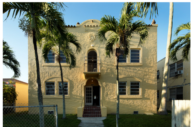
Figure 1.6: A Mediterranean Revival apartment building in Shenandoah (source: ©Steven Brooke Studios, Inc.).
