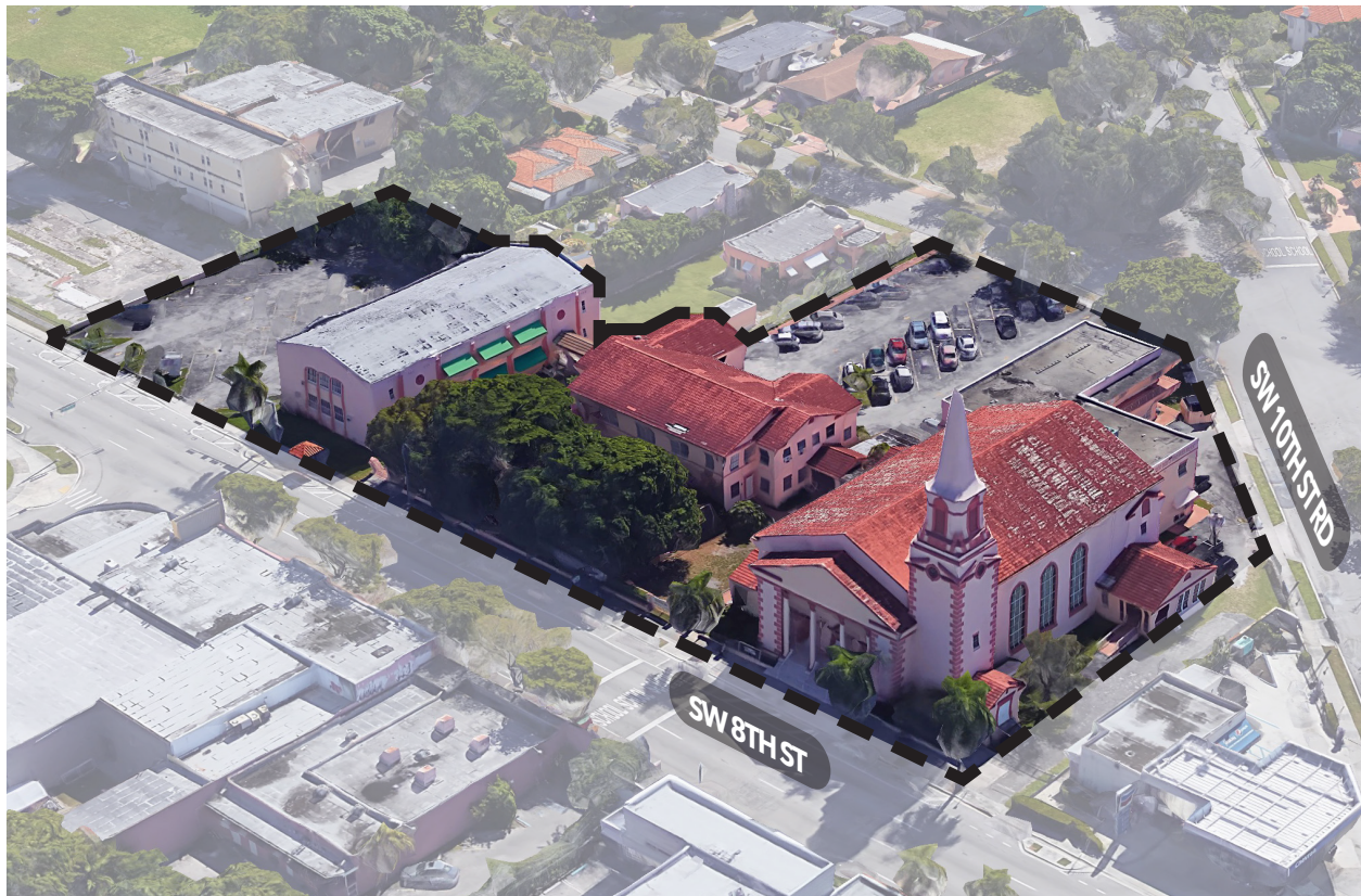
Figure 2.53: Aerial view of the location of Shenandoah Presbyterian Church (source: Google Maps).
