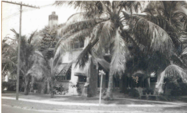
Figure 3.71: This large Mediterranean Revival residence at 1695 SW 11th Street originally had a large landscaped front yard facing SW 17th Avenue (source: City of Miami, Florida Historic Preservation Office Tax Card Photographs).
