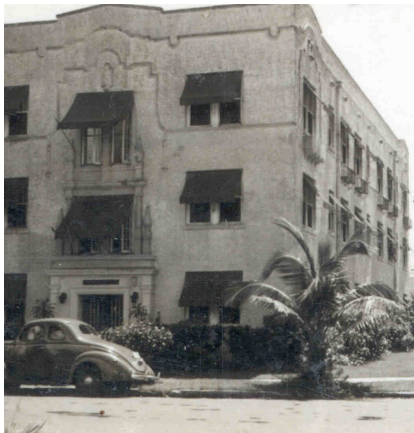
Figure 2.150: Photograph of the building at 829 SW 18th Avenue, designed by architect Ralph A. Preas (source: City of Miami, Florida Historic Preservation Office Tax Card Photographs).
