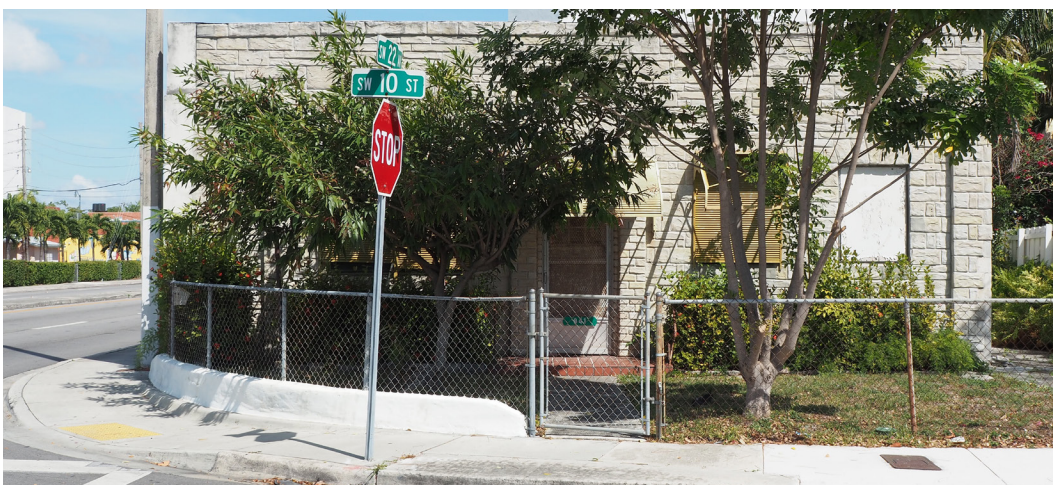
Figure 3.70: Current photograph (2019) of the residence at 941 SW 22nd Street. After road widening on SW 22nd Avenue in the 1970s, the commercial portion of the building was demolished (source: Plusurbia Design).
