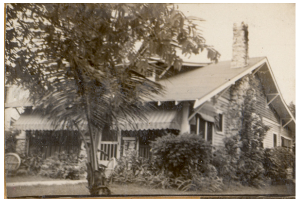
Figure 2.82: Historic photograph of a Bungalow with a porch that has since been enclosed at 820 SW 13th Avenue (source: City of Miami, Florida Historic Preservation Office Tax Card Photographs).
