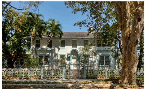
Figure 3.49: Current photograph (2019) of a Colonial Revival residence at 1147 SW 13th Avenue (source: © Steven Brooke Studios, Inc.).
