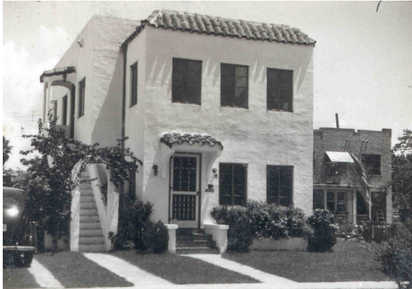
Figure 2.134: Above, a historic photograph of 1841 SW 9th Street residence, one of the 1937 Mediterranean Revival stacked duplexes (source: City of Miami, Florida Historic Preservation Office Tax Card Photographs).
