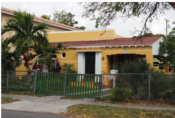
Figure 3.62: Current photograph (2019) of a Streamline Moderne residence at 2129 SW 12th Street (source: Plusurbia Design).
