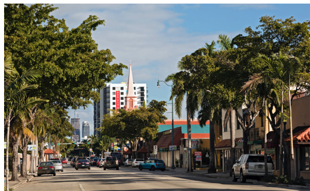
Figure 2.58: The spire of the Neo-Classical Revival Shenandoah Presbyterian Church has served as a memorable icon of the neighborhood that was visible from long distances, marking an entrance to Shenandoah and serving an important place-making role in Shenandoah, Calle Ocho, and Little Havana. This photo of the iconic steeple was taken for the National Trust for Historic Preservation as part of the Little Havana National Treasure effort (source: ©Steven Brooke Studios, Inc.).
