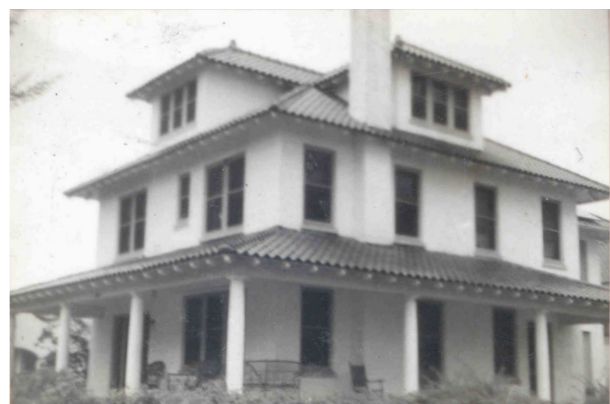
Figure 3.26: Historic tax card photograph of the American Foursquare at 1601 SW 10th Street (source: City of Miami, Florida Historic Preservation Office Tax Card Photographs).
