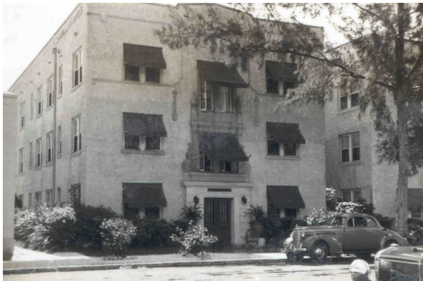
Figure 3.11: Historic tax card photograph of 829 SW 18th Avenue, an example of the kind of Mediterranean Revival center-hall/ walk-up apartment building that are interspersed throughout the neighborhood (source: City of Miami, Florida Historic Preservation Office Tax Card Photographs).
