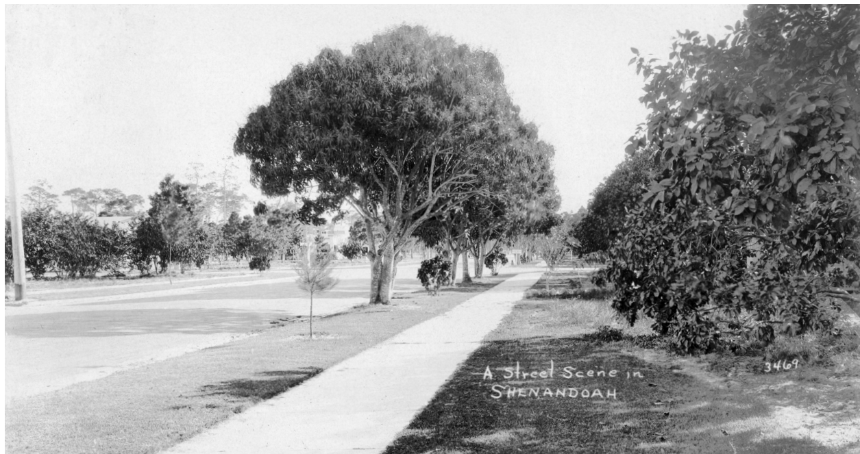
Figure 2.21: Historic photograph of an improved street in Shenandoah prior to construction of residences. Note the presence of the original fruit trees of the Ferris' Grove (source: Matlock Photo Collection, HistoryMiami).
