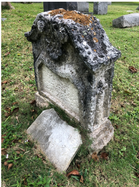
One of the five (5) coral stone (oolitic limestone) markers with its detached marble plaque. This marker should be prioritized when determining overall cemetery treatment priorities due to the uniqueness of the material.
